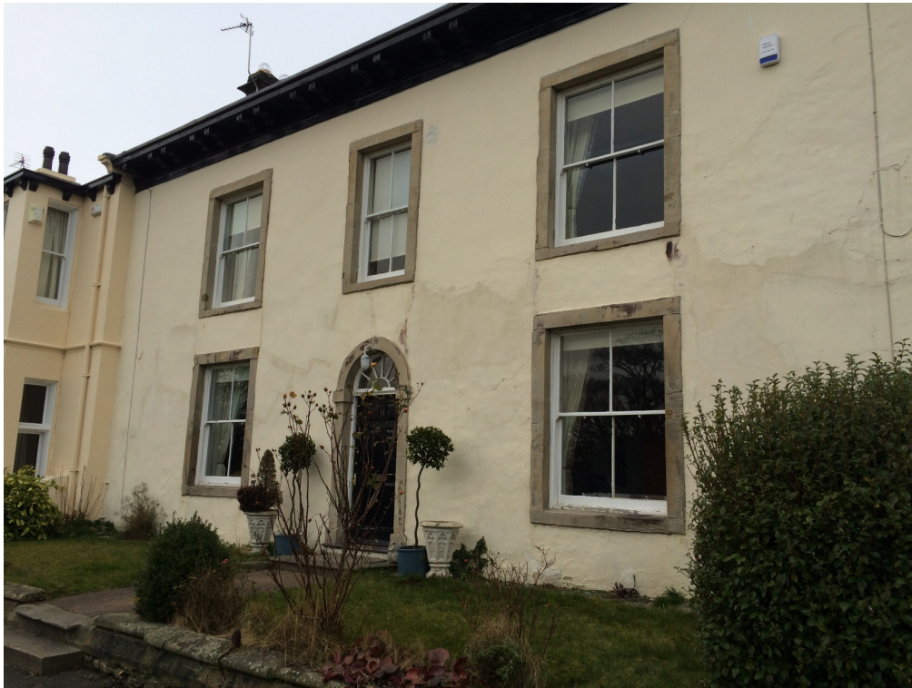
Fig.3 - View of the front / South elevation.
