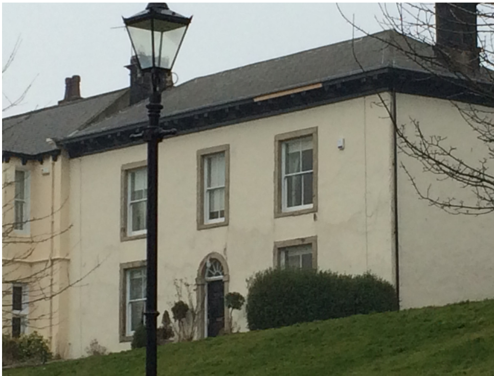
Fig.1 - View of `The Rectory` from Whitburn Front Street.
