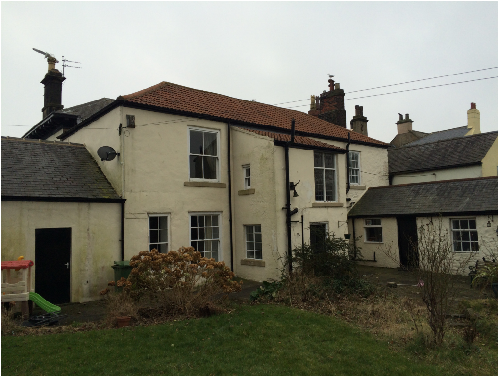
Fig.6 - View to the rear of the property indicating existing windows and red roof tiles to be replaced.
